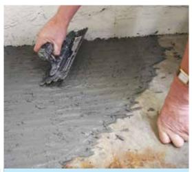
**C** Fix down the Plinth to the floor using a full bed of flexible cement based tile adhesive. Use the adhesive to help level any uneven floors.
