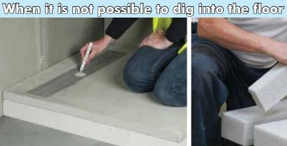
A The 100mm thick plinth will encase the drain and supper the Showerlay.
