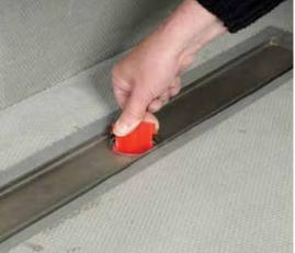
**10** Screw the flange ring through the Showerlay into the drain below. Hand-tighten using the red "key". No sealants should be used.
