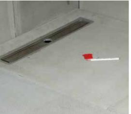
**11** Showerlay-Linear are 40mm thick. The rest of the floor can be raised to this height using Multiboard 40mm.
