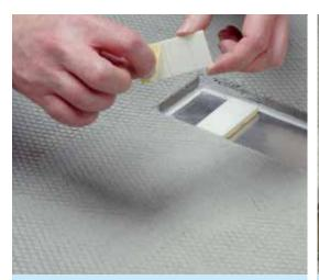
**9** If the height needs to be increased further, additional 2mm thick spacers can be stuck on top of the other spacers.
