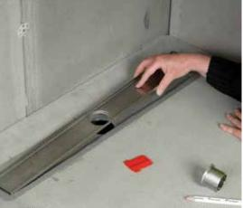
Using a cement-based flexible tile adhesive, stick the Showerlay to the floor and position the drain tray into position (there is no need to secure this with adhesive).
