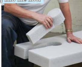
**B** Cut out a hole for the gully (diameter 130mm – 150mm) and a channel for the drain pipe.
