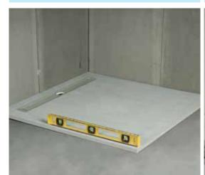
Check that in position, the Showerlay is on a flat surface offering support – especially around the drain.
