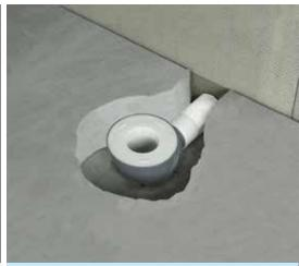
Solvent weld the drain to the BS40mm pipe so it is positioned centrally in the hole.
